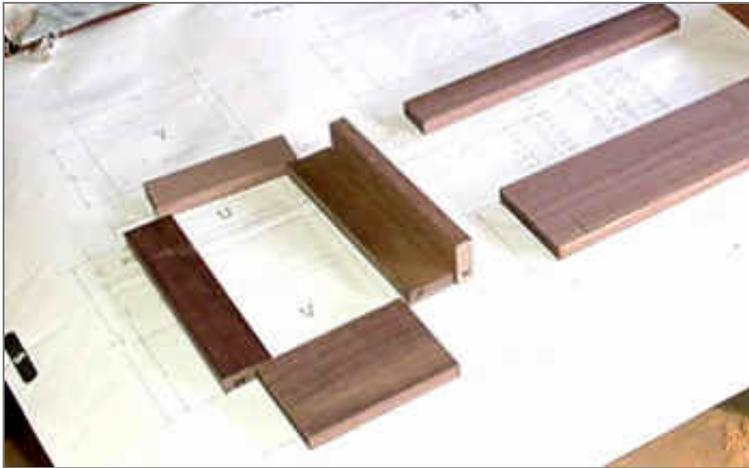
This is what I am working on. The "L" on the right is made up of the two stiles I just profiled with the locking miter bit.
