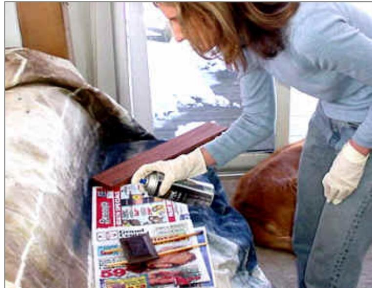
In between coats of the polyurethane, Beth sands the veneered, flat areas with a sanding block and 220 grit paper. She follows this with a piece of the paper rolled up to smooth the MDF edges.
